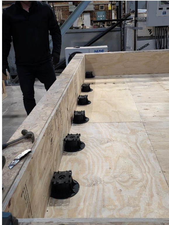
Plate 1 – Pedestals Positioned at 600 mm Centres
