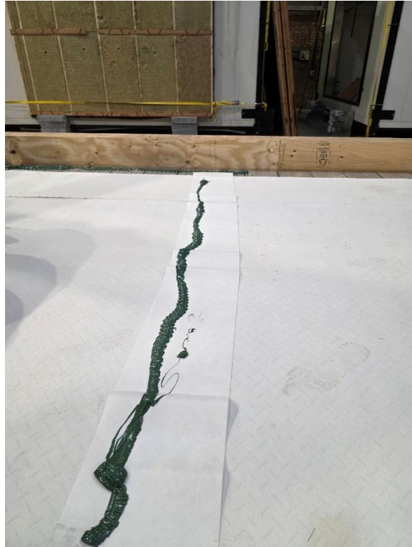
Plate 6 – Adhesive on Jointing Strip for the Artificial Grass
