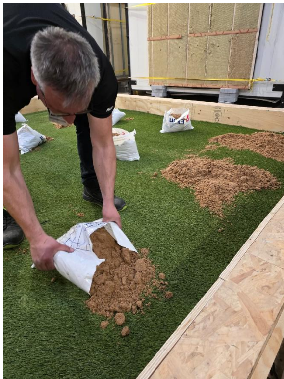
Plate 9 – Grass Fully Installed, Sand is Laid Out on the Surface
