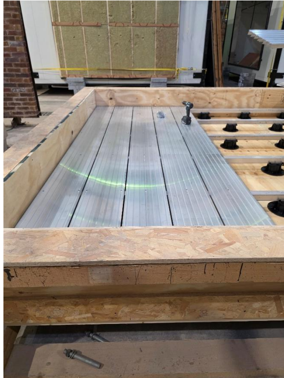
Plate 5 – 6-8 mm Gap Left Between Each Base Board
