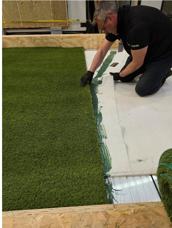
Plate 8 – First Half of the Artificial Grass Installed with Joint Adhered to the Underside of the Grass
