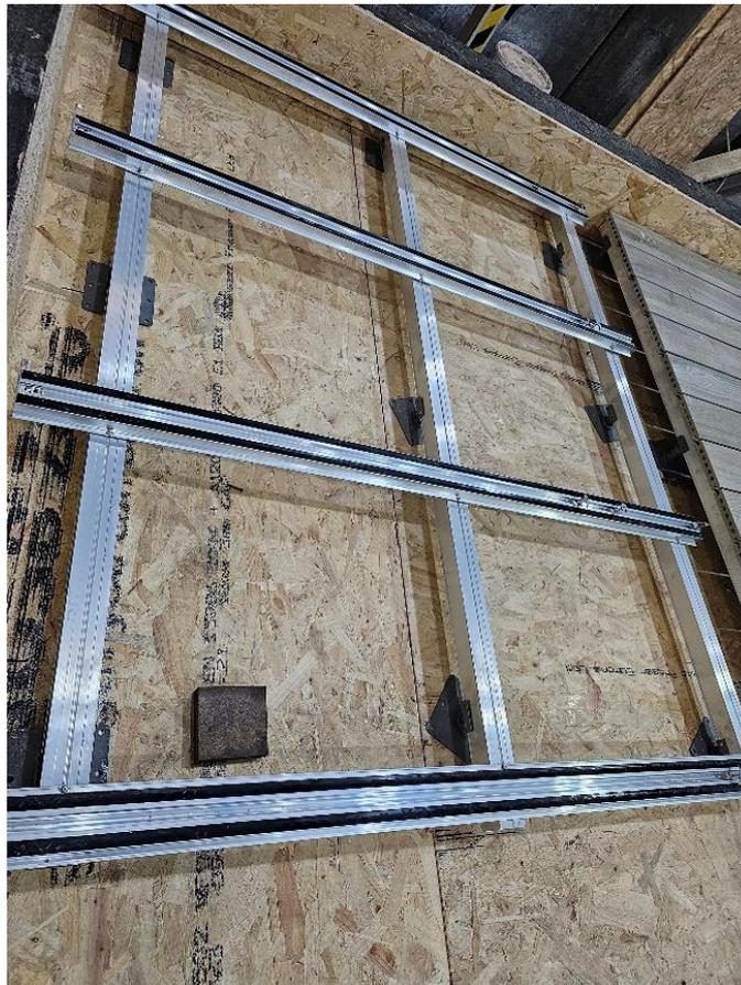
**Plate 18** – Rails Attached with a Screw into Each Joist
