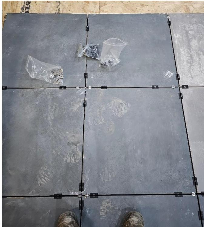
**Plate 21** – Rails and Visual Fix Test Sample Fixed in Place
