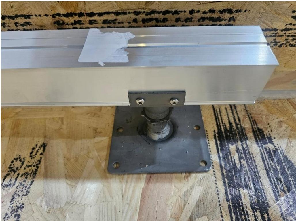
**Plate 10** – Pedestals Screwed to Joists
