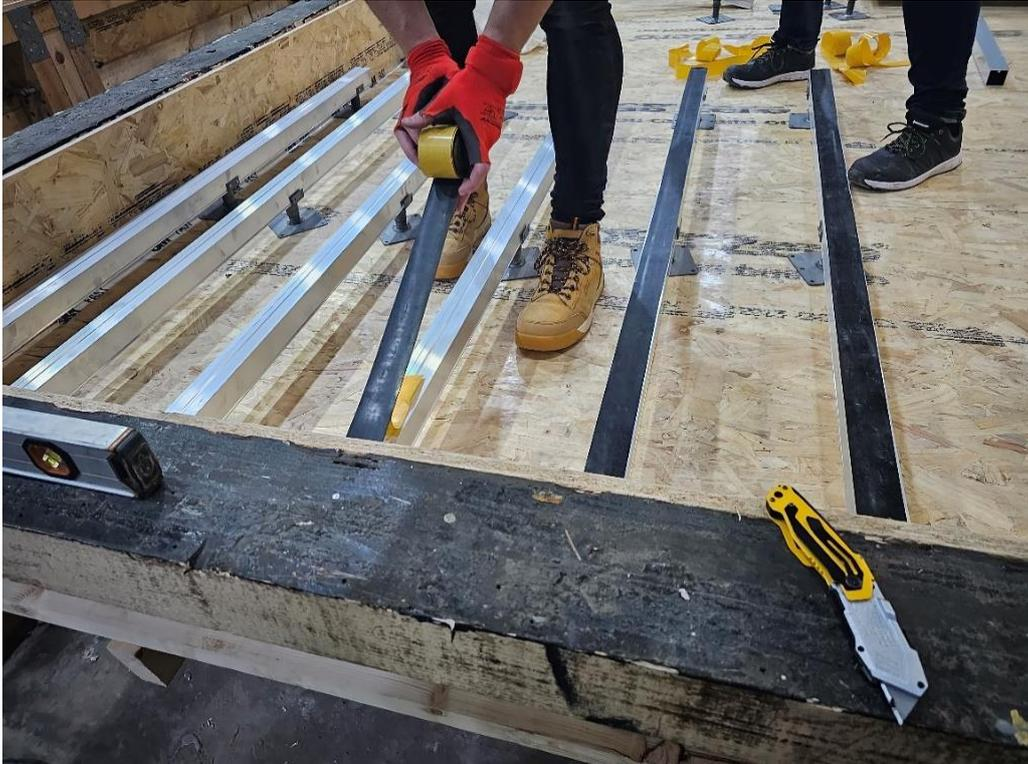
**Plate 9** – EPDM Applied to Joists
